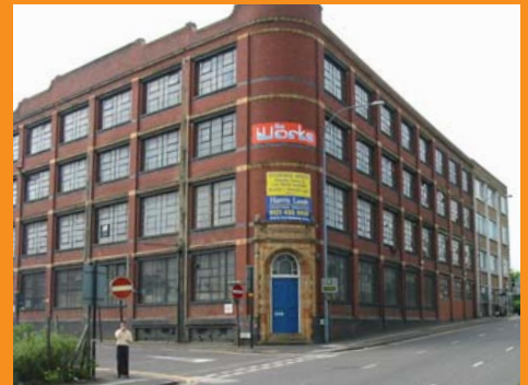
St Georges Works Building on Pope Street.
